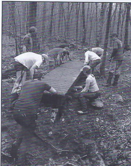
Moving a bridge at Wilton Woods. Photo by John Sweeney
